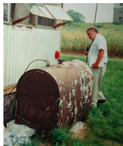
CHECK TANK AND PIPE FOR UNSAFE CONDITIONS
