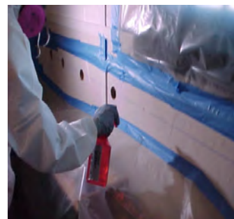
FIG. E-13: WET MIST AND WIPE ALL SURFACES
