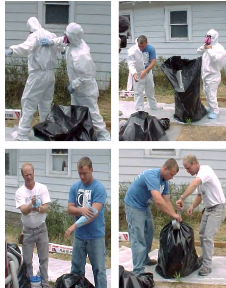
FIG. E-21: FINAL PERSONAL CLEANING
