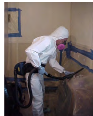
FIG. E-12: HEPA VACUUM ALL SURFACES
