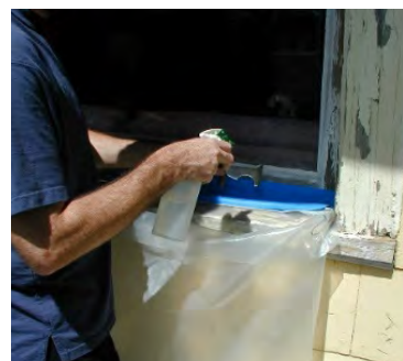
FIG. E-8: USING A CATCH BAG AND WET MISTING
