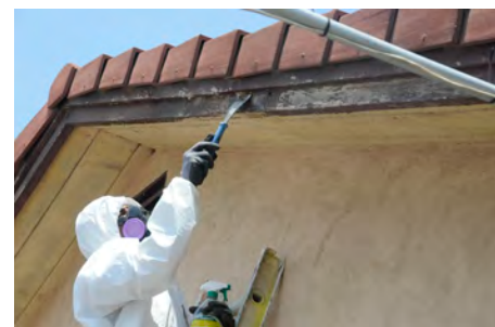
FIG. G-4: LEAD-SAFE WEATHERIZATION
