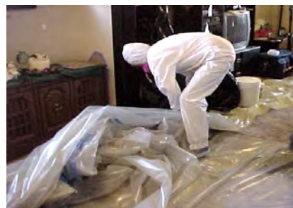
FIG. E-17: REMOVING INTERIOR POLY
