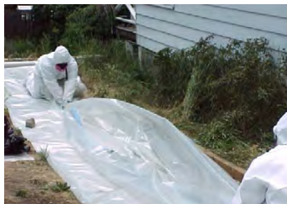
FIG. E-18: REMOVING POLY GROUND COVER
