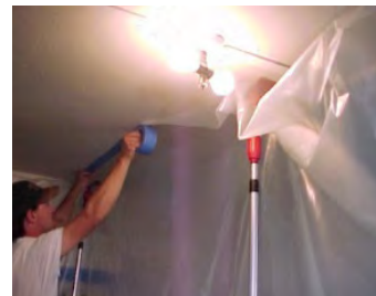
FIG. E-4: SEALING A BARRIER WALL
